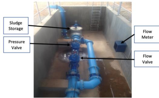
Figure 60 – Installed PRV1
